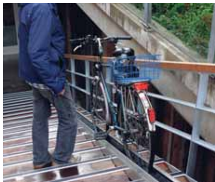
Borstelgoot in stalling Paradiso
